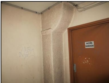
Photo N° 930 AMIANTE CIMENT -- DEGAGEMENT -1 Gaines & coffres verticaux Ventilation haute (Fibres- ciment)
